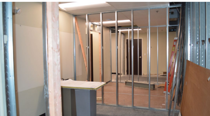
New office space is constructed at the Township.
