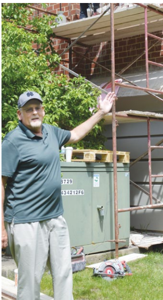
Supervisor Heneghan observes gym expansion construction.
